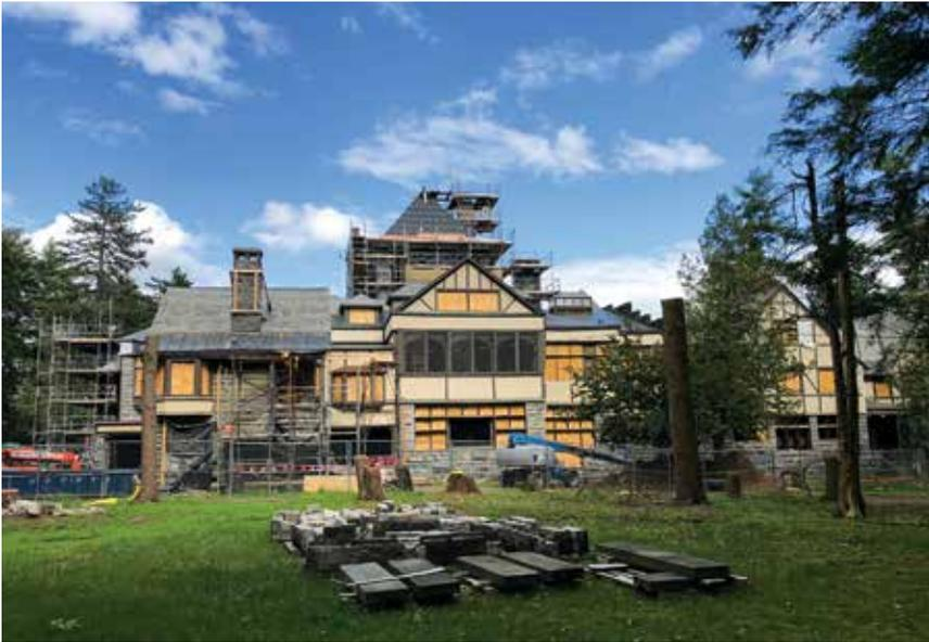
▲ To stabilize the porte-cochère, the chimney above Spencer's wing has been buttressed, while the stairwell is dismantled, with limestone pieces organized for reassembly.
